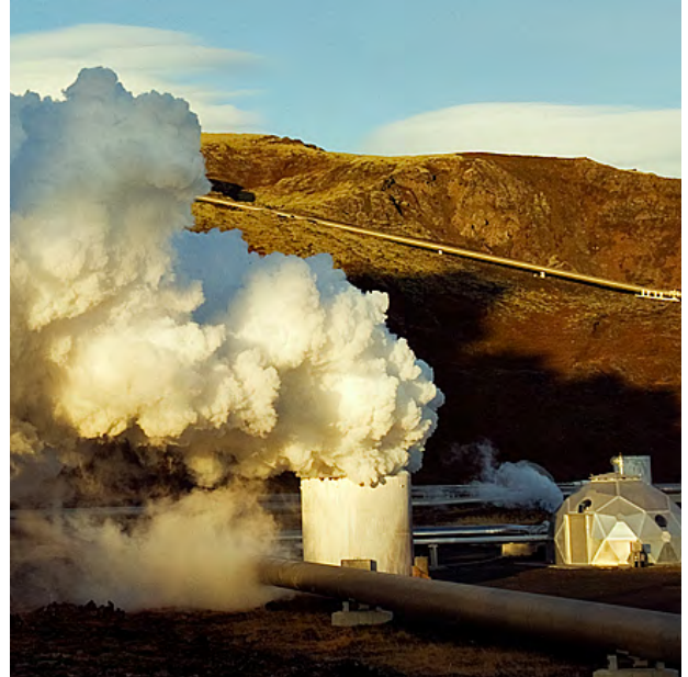
▲ Geothermal Power Plant in Iceland
